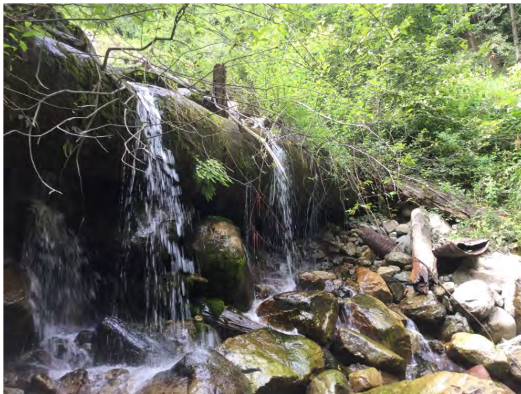
Large log retaining fill at outlet
