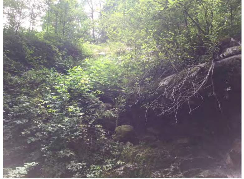
Large log retaining fill at outlet
